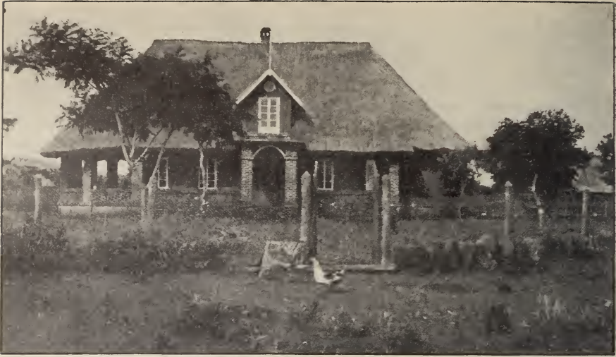
WHERE THE TOUR STARTS The mission residence at Ochileso
